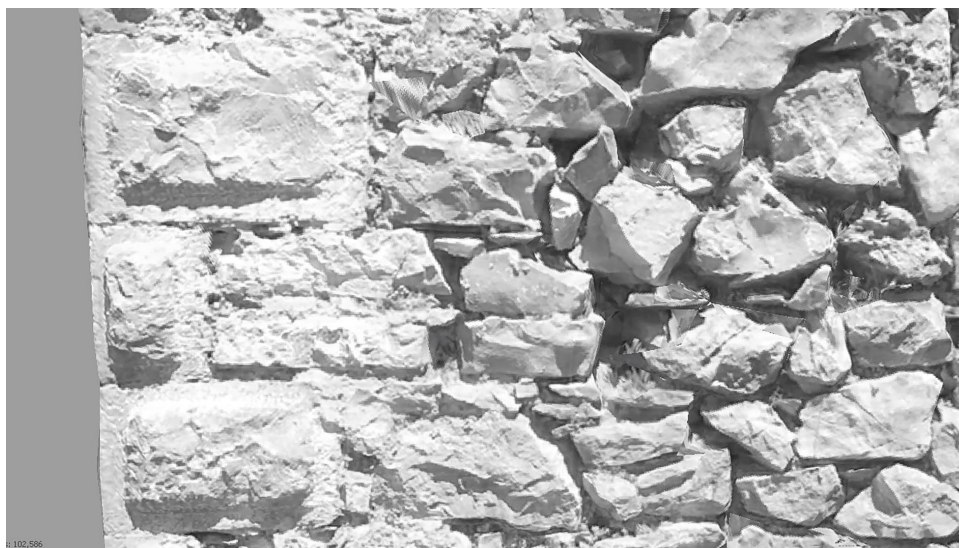
Figure 7. Screenshot showing reconstructed wall of Building 84 generated from frames extracted from iPad videos.
