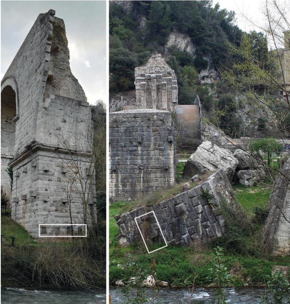
Figure 8. Holes in first and second pylon.
