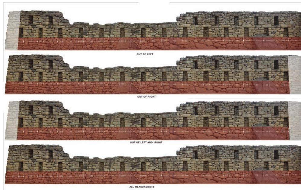
Figure 3. The four models of niches layout execution.
