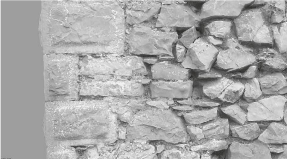
**Figure 6.** Screenshot showing reconstructed wall of Building 84 generated from DSLR photographs.
