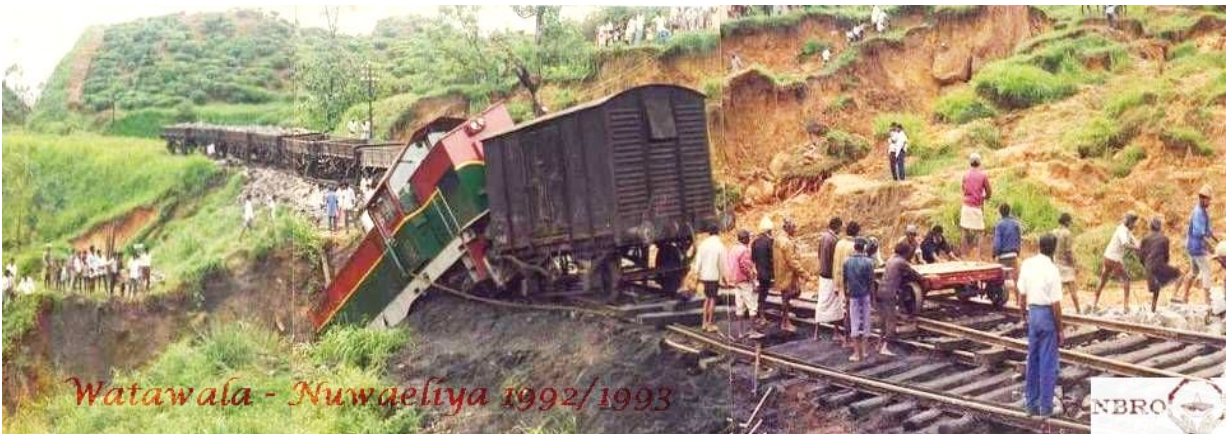
(d) Watawala landslide which damaged major railway line – 1992/1993
