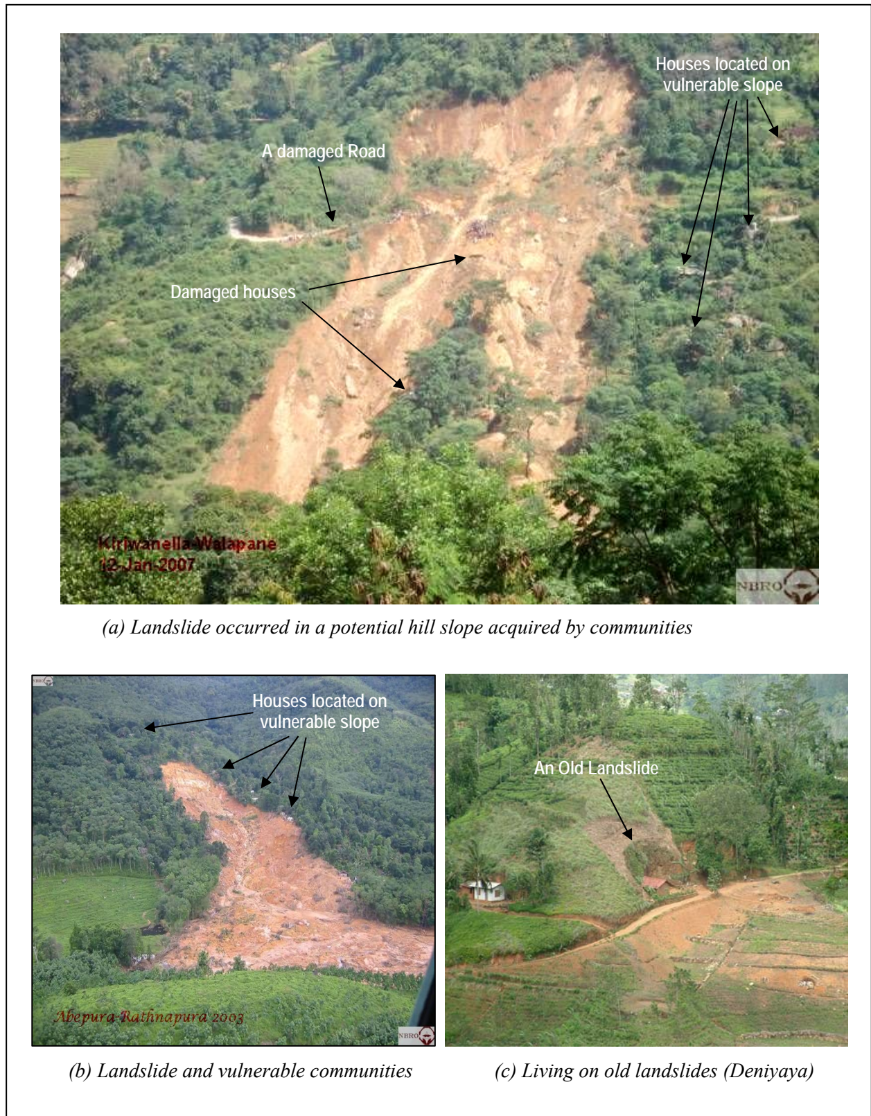
Figure 4.3: Human intervention into vulnerable hill slopes and landslide disaster in Sri Lanka: (a) Kiriwanaella, Walapane landslide in which 12 people were killed and 5 houses were buried - Jan. 2007; (b) Elapatha, Abepura-Rathnapura landslide occurred on 17 th May 2003 killing 67 people.
