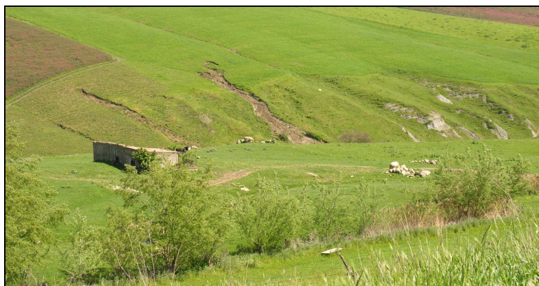
Figure 5.14. Landslides located in the upper part of the San Giorgio River basin (10.04.2011).
