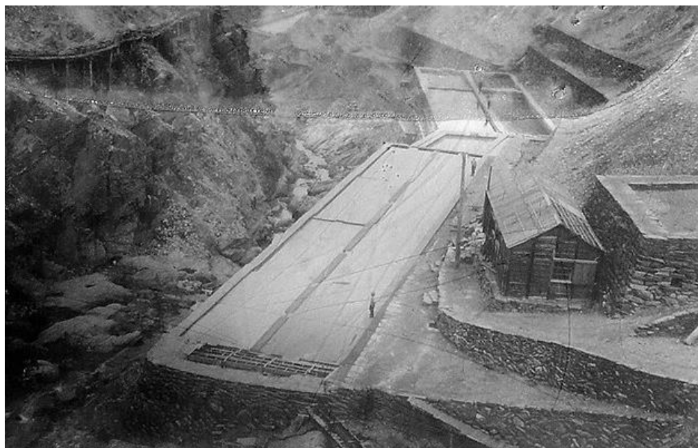
Fig. 53: Basins for wet copper production at the Besshi mine in Shikoku, where wet copper production was first initiated in 1875.
