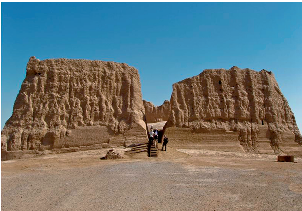
Fig. 7. The Greater Kyz Kala monument, showing a metal staircase inserted through an erosion hole in north wall in Spring 2007.
