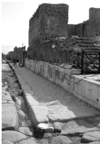
Figure 13. The north side of the Tempio della Fortuna Augusta showing a length of sidewalk devoid of sidewalk holes.
