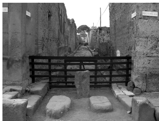
Figure 14. South end of the Vico del Labirinto blocked to cart traffic by an upright stone.
