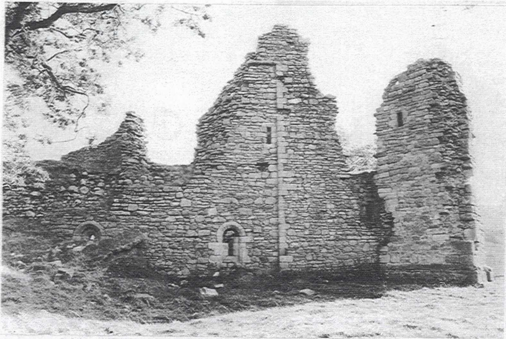
Figure 35.1: View of the west elevation, west face.
