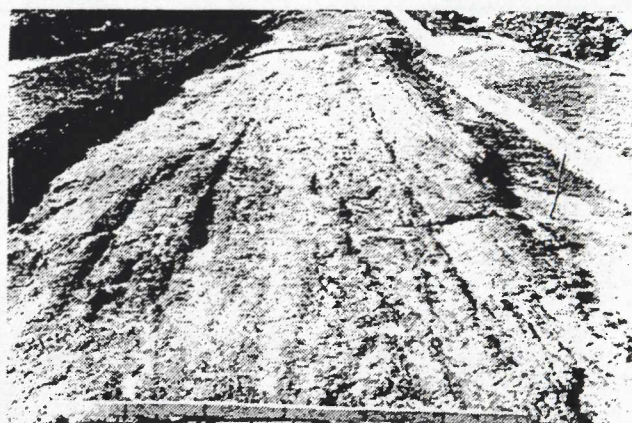
Figure 16.3: Metalling of Roman slag on the London-Lewes road at Holtje (Margary 1940).
